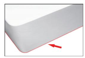
Allow silicone to cure for 24 hours before using tub.
