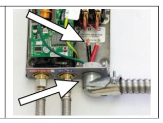
**2.** The power leads are to be secured to the L1 and L2 or L and N connectors on the terminal block or relay. The ground lead is to be secured to the GND connector on the block or the green ground wire with the provided wire nut.
