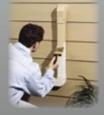
DiversiTech recommends attaching the base to the wall or ceiling and the line sets to the system every 15" to allow for the system to carry the full weight of the line sets.
