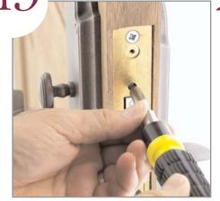
Tighten the cylinder set screw by turning clockwise. **Do not over tighten. Do not use a power screw driver.**
