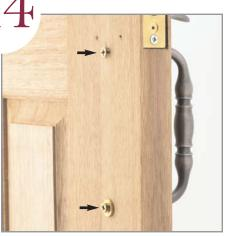
Start the thru-bolts which will hold the exterior trim. (Use screw cover washer under the bottom thru-bolt.) Tighten both securely.
