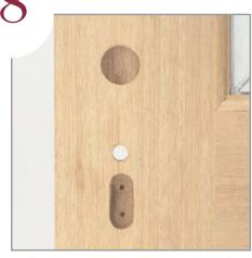
Drill appropriate holes as indicated on yellow lock template. **DO NOT OVERSIZE HOLES.** Only top two holes are drilled for knob to knob and lever to lever sets.
