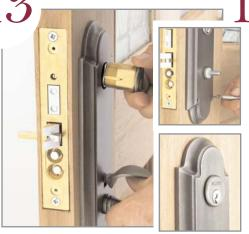
Place the cylinder through the trim. Partially insert key into cylinder. Thread the cylinder into the lock until it is against the trim and Baldwin name is horizontal. For knob to knob and lever to lever sets - Install aligning bushing and fasten trim with supplied screws. Remove bushing - go to step 16.
