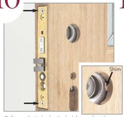
Drill two pilot holes for the lock face, adjust the bevel and install the lock. Shim between the lock and door on cylinder side as shown to prohibit the cylinder from pulling the lock case off center. (Failure to shim the lock may cause the cylinder to sit unevenly on the surface of the trim.)
