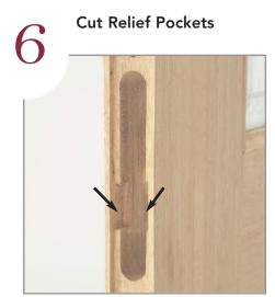
Cut the relief pockets 3/8" deep on both sides for the Latch Hinge, 2-1/2" and 2-3/4" backset only. (Does not apply for 1" front.)
